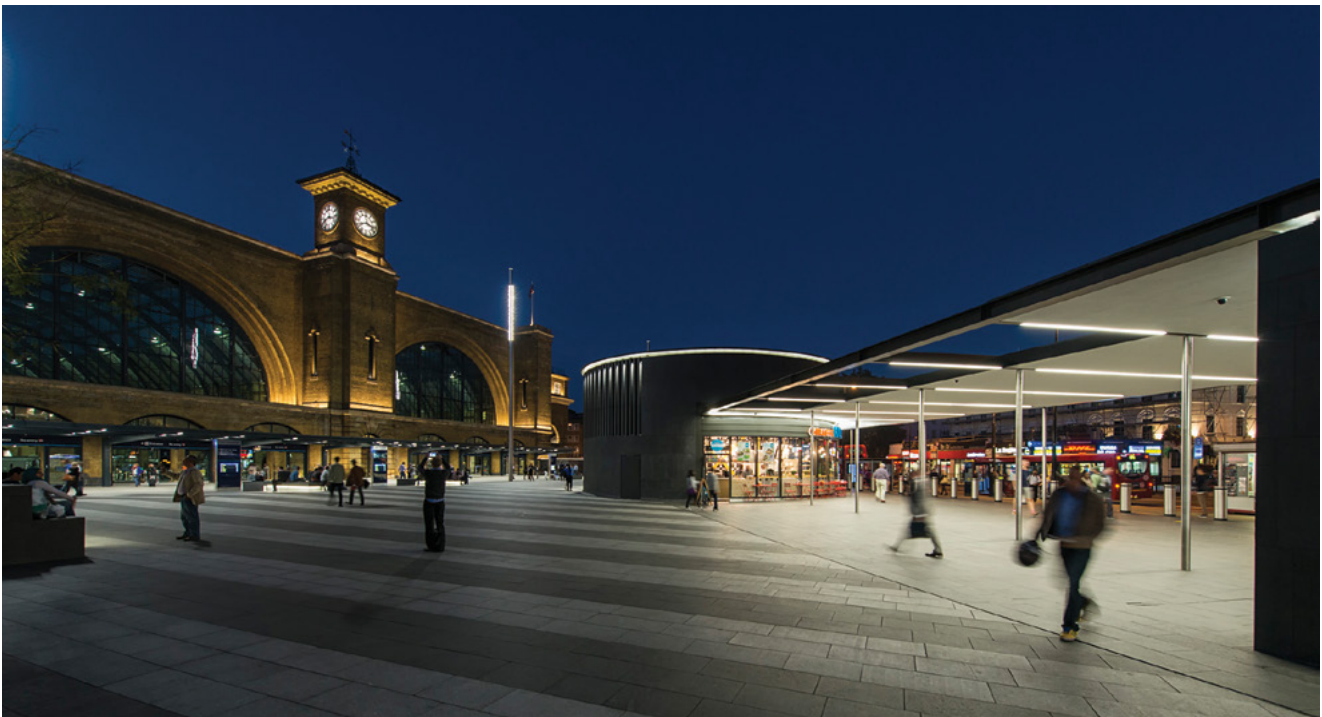
Kings Cross Square | London, UK Lighting Design by studioFRACTAL Lighting Design | Photography © Will Scott Photography
